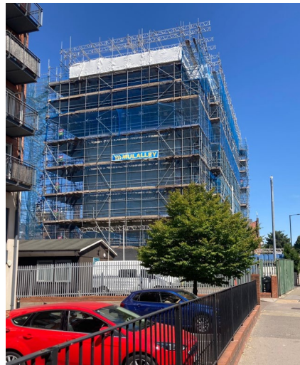
White Sheeting removed
