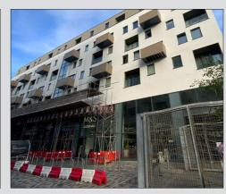
• Elevation D, CC and E have scaffolding removed from level 6-5. The remaining levels 4-1 are progressing, we expect to complete the render by end of December assuming the cold weather permits this. Any remaining scaffold will be down early in the New Year.
